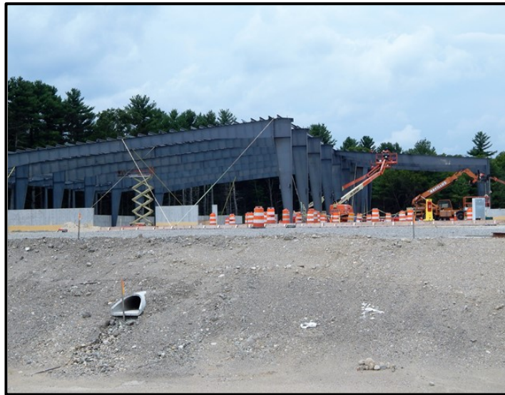
Steel Erection Progress
