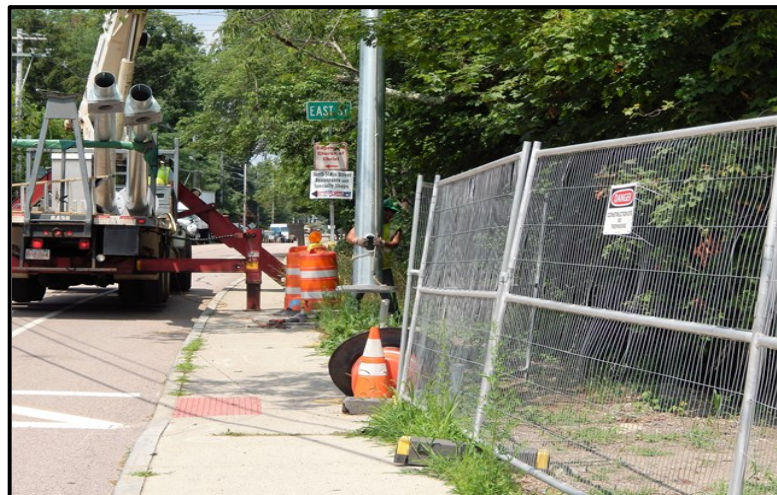
Contractor Placing Traffic Signal Poles
