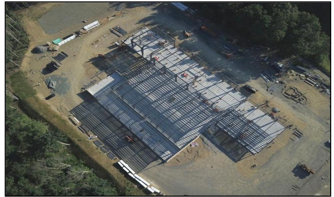
Drone Aerial View of the Site and Structural Steel Work
