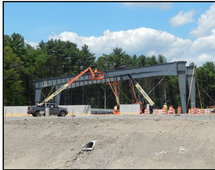
Steel Erection Has Begun for the DPW Building
