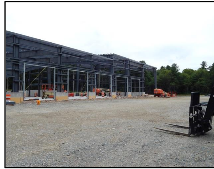
Overhead Door Frames Installed
