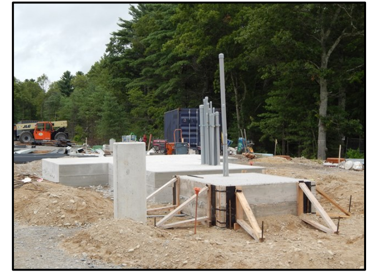
New DPW Generator Pad Installed
