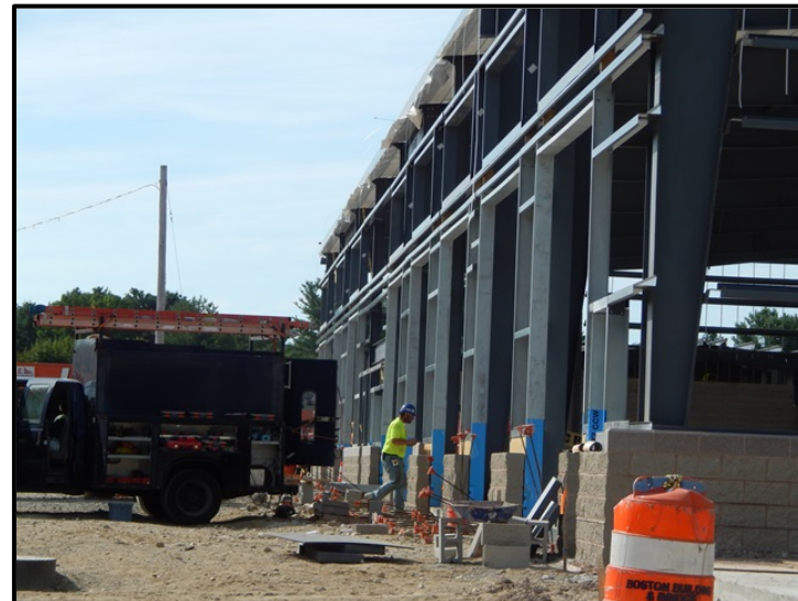
Exterior CMU Work Continues Around the Superstructure.
