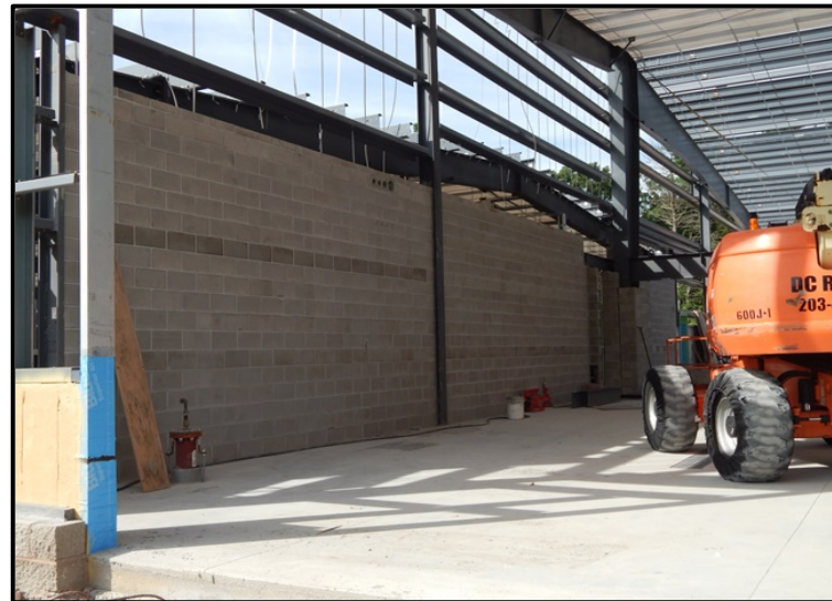
Interior Concrete Masonry Unit (CMU) Work in the Admin Area.
