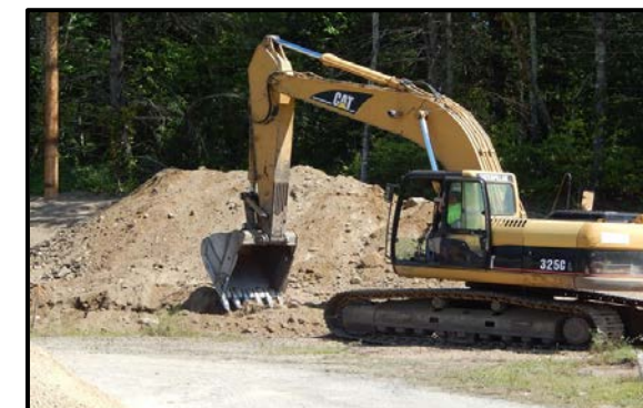
Excavation for Waterline & Hydrant Relocation at Fish & Game.
