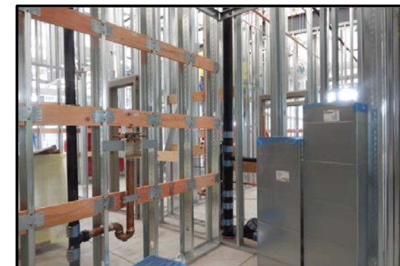
Interior Metal Stud Framing, Duct Work & Piping In Admin Area.
