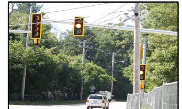
Traffic Signals Operational on East Street.
