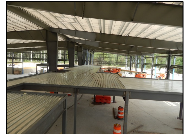
Mezzanine Structure Installation.
