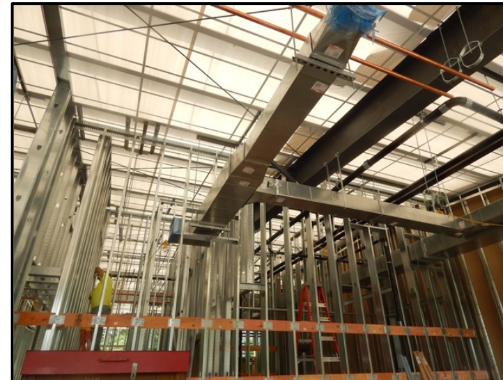
Interior Metal Stud Framing and Duct Work Installation.
