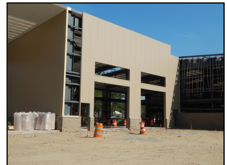
Siding Installed at the Knock Down Pad and Equipment Bays.
