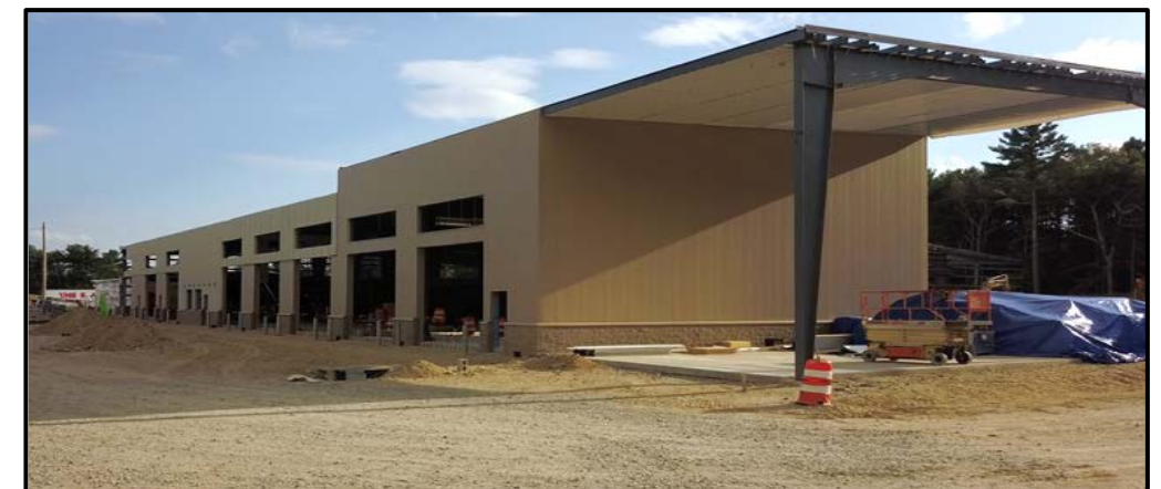
Siding Installed at the Knock Down Pad and Equipment Bays.
