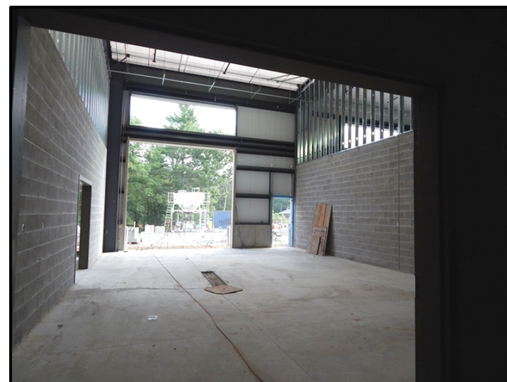
New Vehicle Bay - Masonry Work.
