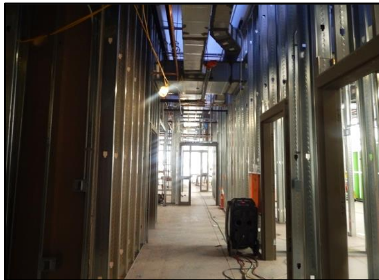
Metal Framing in Admin Area. Door Frames Established.
