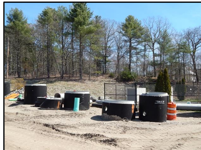
Sewer Piping for Underground Installation at East Side of the Site
