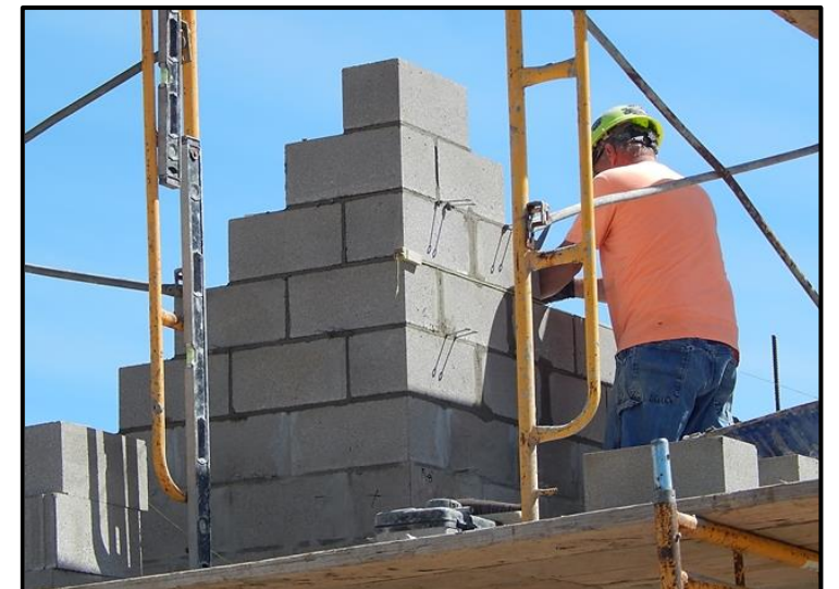
Mason at Work at Building A Cellblock
