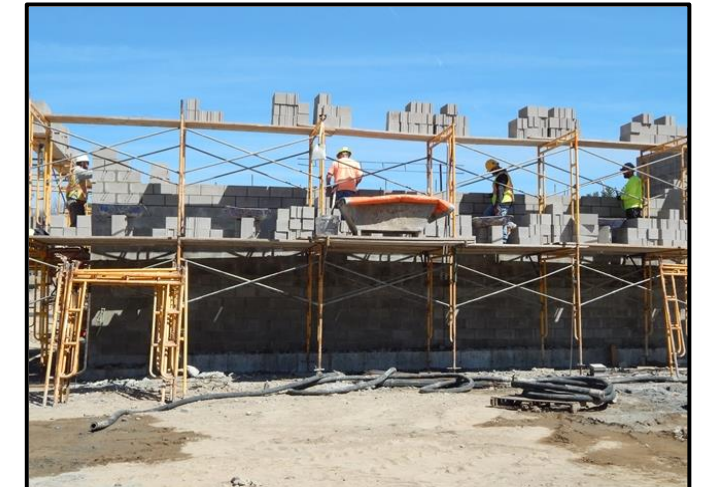
Masonry Contractors Progressing with Cell Block CMU
