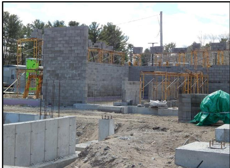
Cellblock Masonry Work in Building A Area Underway - PS
