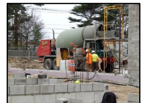
Grout Delivery for Masons
