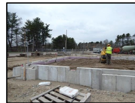
Contractor Utilizing Vibratory Roller for Soil Compaction
