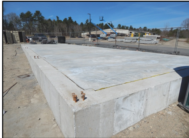
PS Storage Building Slab Complete & Ready for Structural Steel
