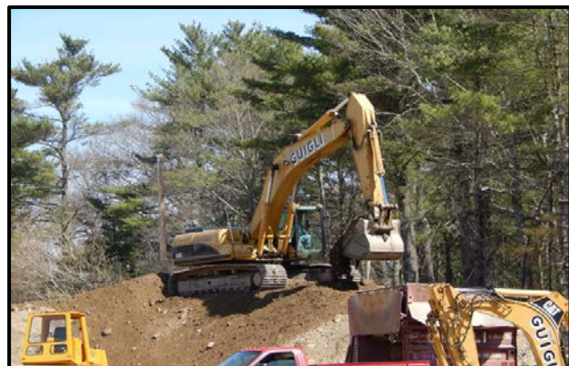
Contractor Screening Gravel for Reuse Onsite
