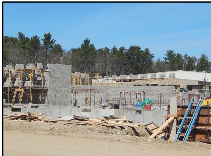
East to West Perspective of Masonry Work at Building A
