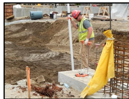
Exploratory Excavation to Record Undocumented Fill
